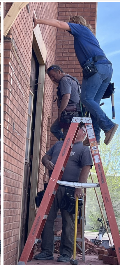
Removing exterior bricks to open entrance from the hall way from the Social Hall into the Commercial Kitchen.
