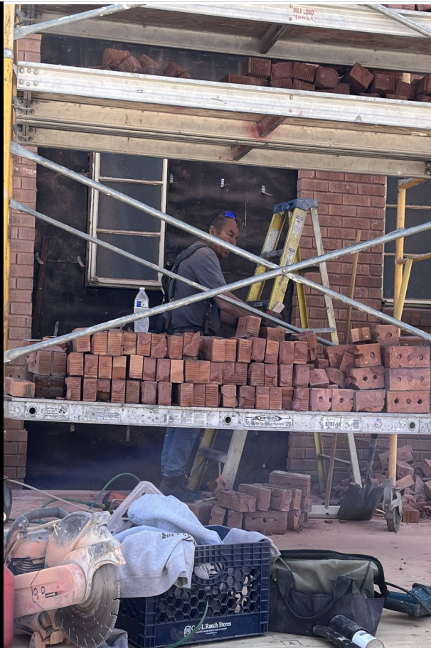
Removing exterior bricks to open entrance from the hall way from the Social Hall into the Commercial Kitchen.
